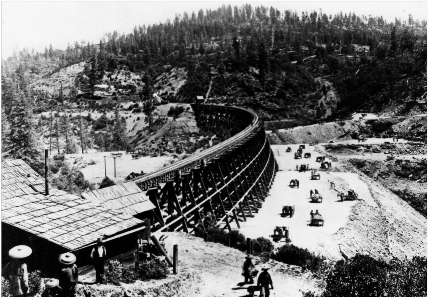
Chinese laborers working at the Secret Town, California, railroad trestle that was built by the Central Pacific Railroad, 1868. From the collection of Pat Jones.
